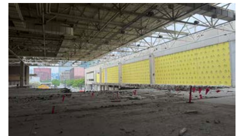
Hall D interiors slab demolition
