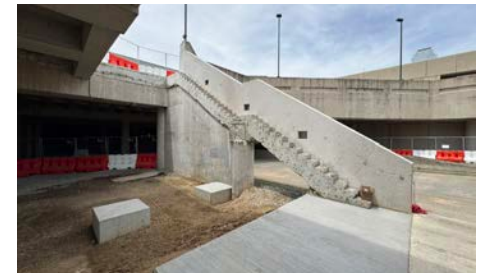
Truck ramp stair preparation
