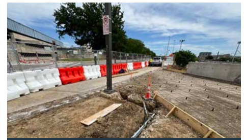
Truck ramp approach slab
