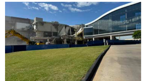
Hall D demolition, view from the Omni
