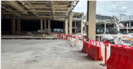
Barrier control during demolition
