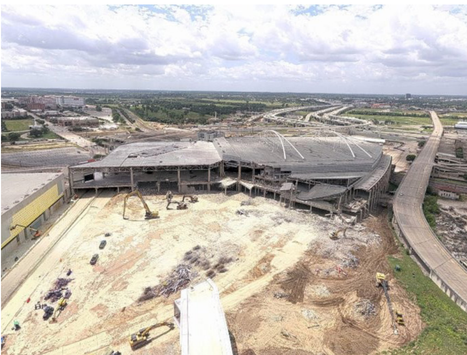
Demolition from North
