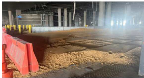
Hall D Demolition
