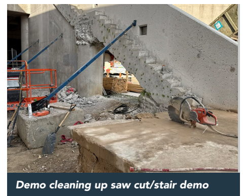
Hall D Demolition
