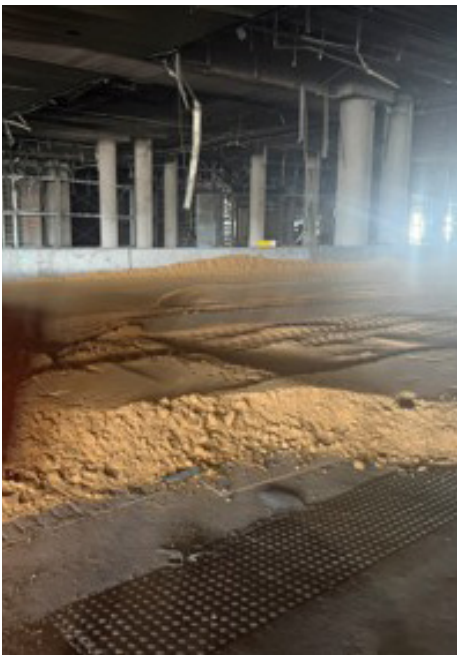
Hall D Demolition
