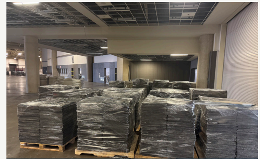
Carpet and ceiling tile ready for Circularity
